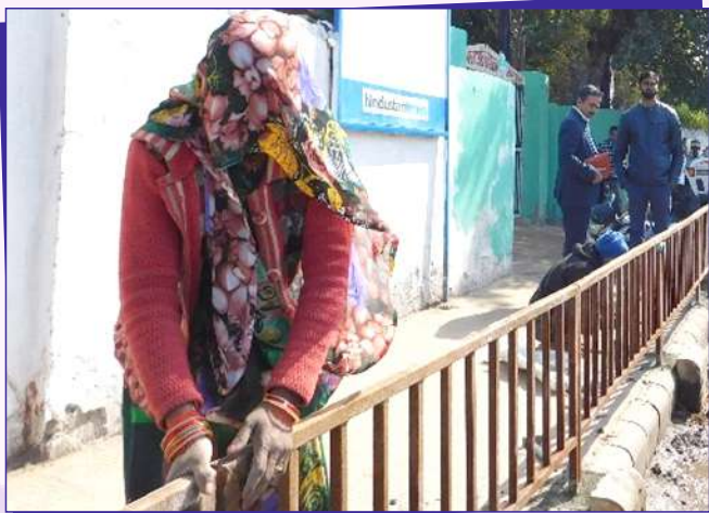
Fencing of footpath at G.B.S school, Civil Lines Gurugram
