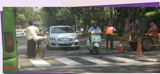
Repainting of Zebra Crossings under Safe School Zone
