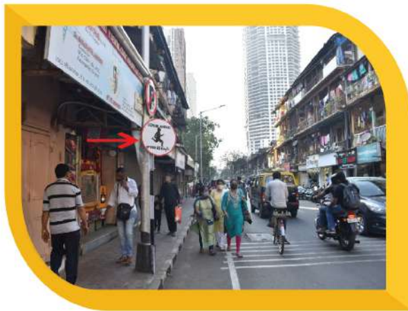
Installation Of Cautionary 'School Sign' And 'No Parking' Signs
