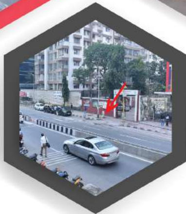
Construction of 'Ramp' for Smooth Walkability of Pedestrians
