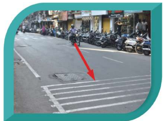
Implementation of Rumble Strips
