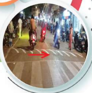
Construction of 'Speed Breaker'
