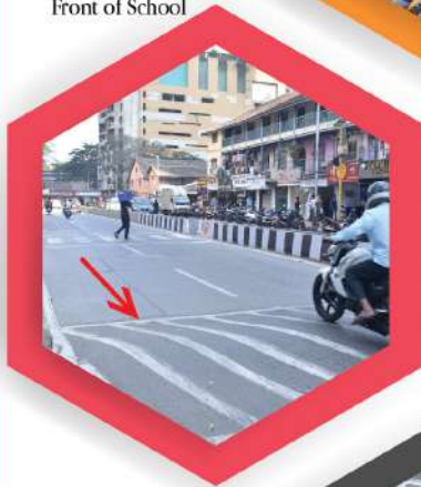
Construction of Speed Breaker as Speed Calming Measures In Front of School
