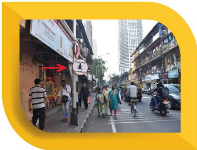
Installation Of Cautionary School Sign And No Parking Board
